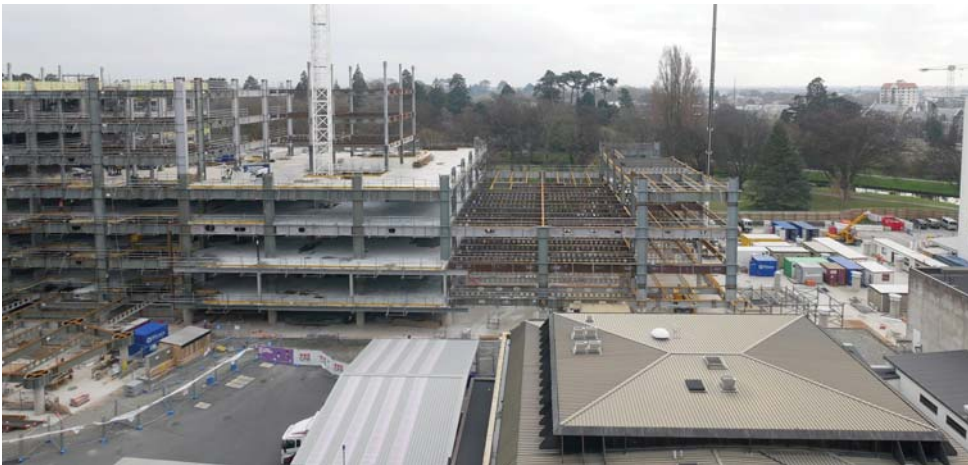
This wide angle shot of the ASB shows the west tower (on the left) with the steel framing up to Level 6, the central core that stays at 3 storeys and the framing on the east tower with preparations underway for the first of several concrete pours that will form the floors of the tower.
